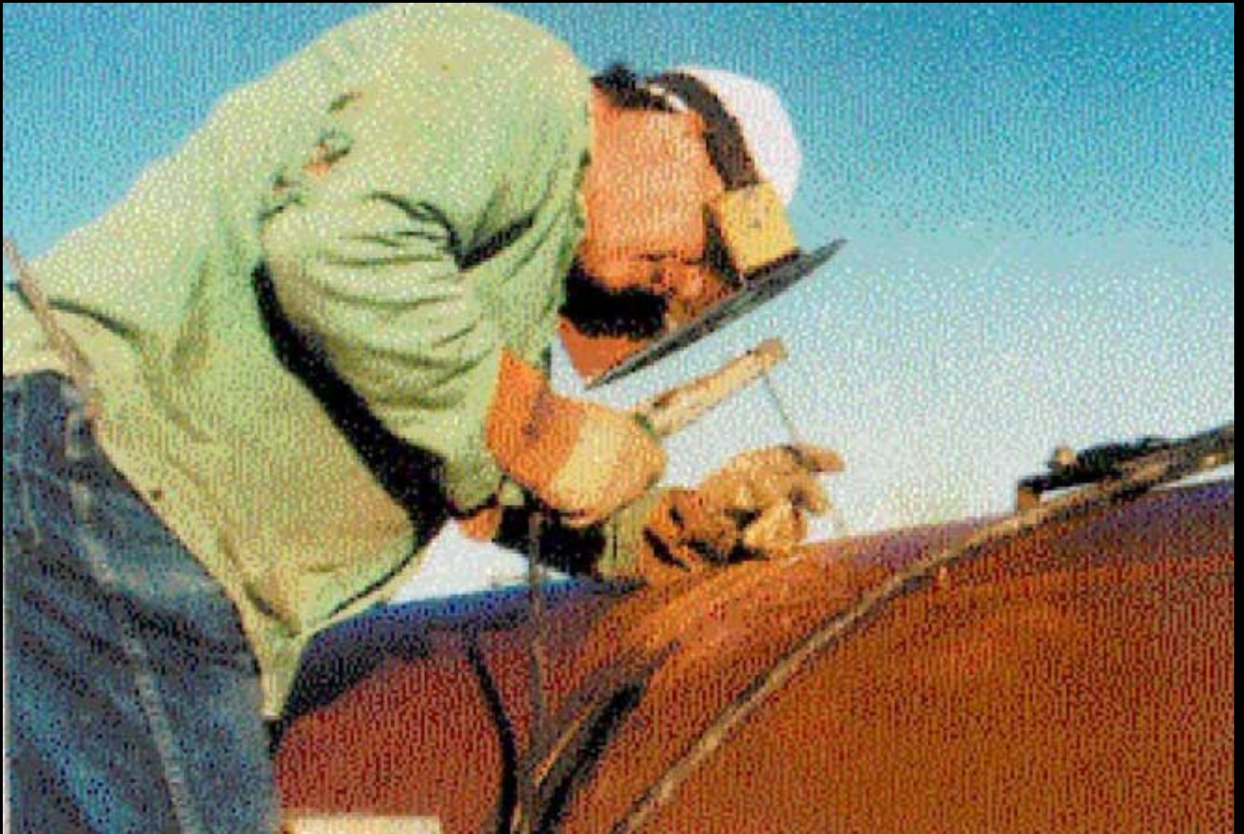
Stick welder joins sections of oil pipe in Alaska.
